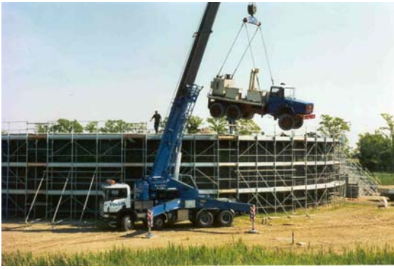
(a) Test embankment. Penetrometer truck for testing after construction.
