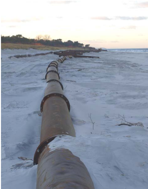
Figure 10. Pipeline for sand fill transport.
