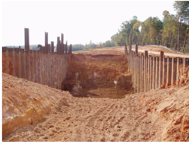
Figure 9 Excavation complete at 6.1m
