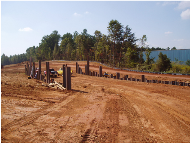
Figure 8 Installed sheet piles
