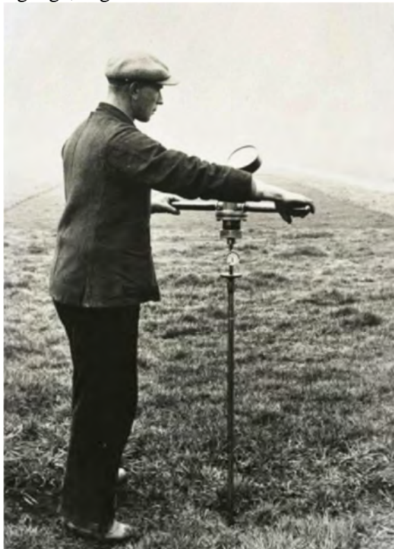
a) Mechanical cone testing around 1950
